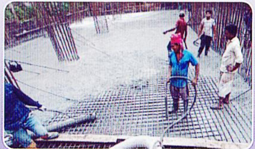
Concreting at site
