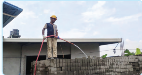
Curing of Block
